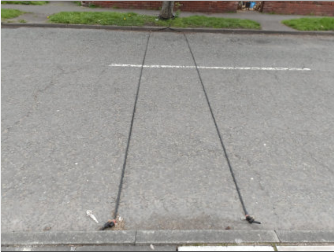
Monitoring equipment on Gosforth Terrace
