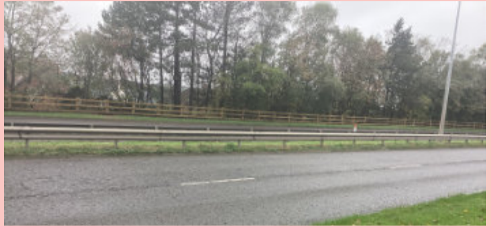
Section of the new barrier on the Felling Bypass
